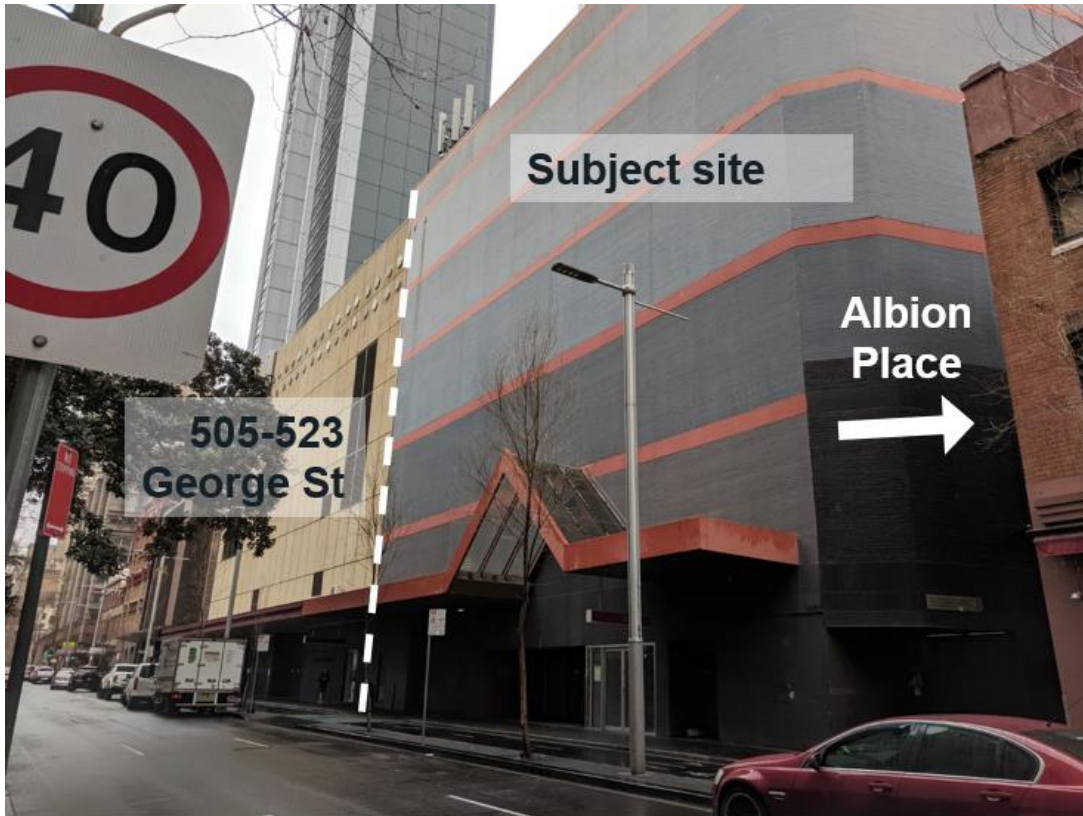
Figure 7: View of site looking northeast from Kent Street
