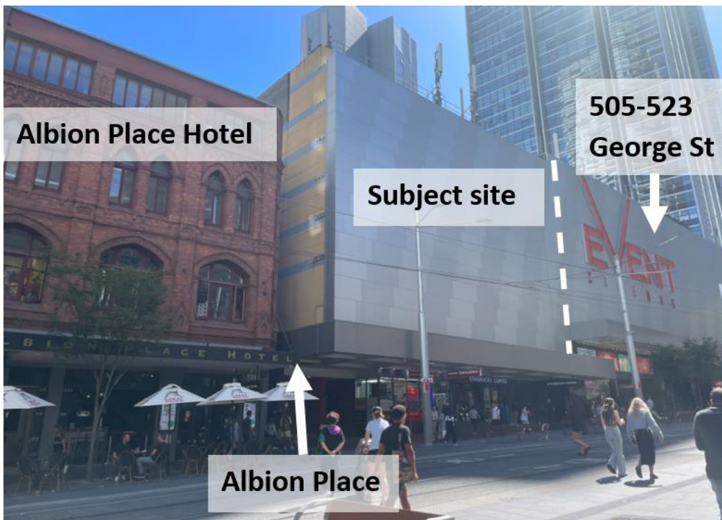
Figure 2: Site viewed from George Street
